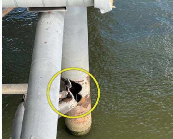
Damage to pier (circled). Left to right: A vertical piling. Insulated pipe, pier support bracing, and railing.
