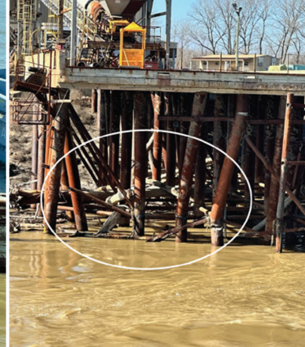
Left to right: The damage to barge ACBL2549 after the contact (circled), and the damage to the Port of West Memphis dock (circled). SOURCE: COAST GUARD.
