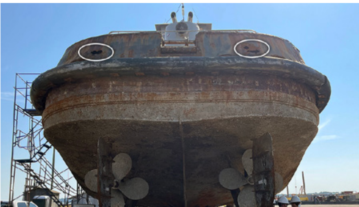
Wastage holes (circled) on outboard plating of stern bulwarks.
