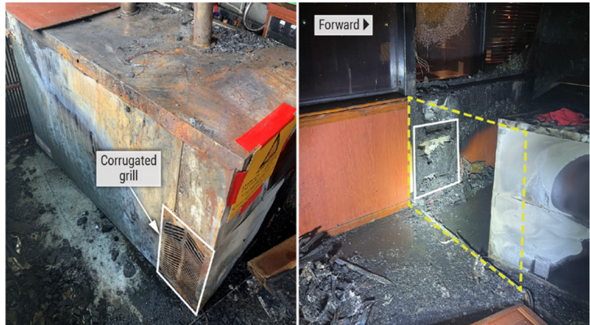
Left to right: Origin area of the fire on corrugated grill (outlined) on main deck bar refrigeration unit, with fire pattern mirrored (outlined) on portside bulkhead. The area of a cabinet end panel in place prior to the fire is indicated by a dashed line. SOURCE: FLORIDA BUREAU OF FIRE, ARSON, AND EXPLOSIVES.
