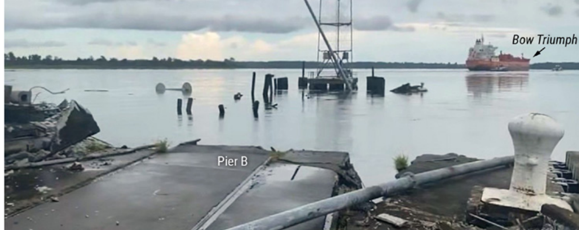
Witness photograph taken shortly after the contact showing damage to Pier B. BACKGROUND SOURCE: JACOB WALL.
