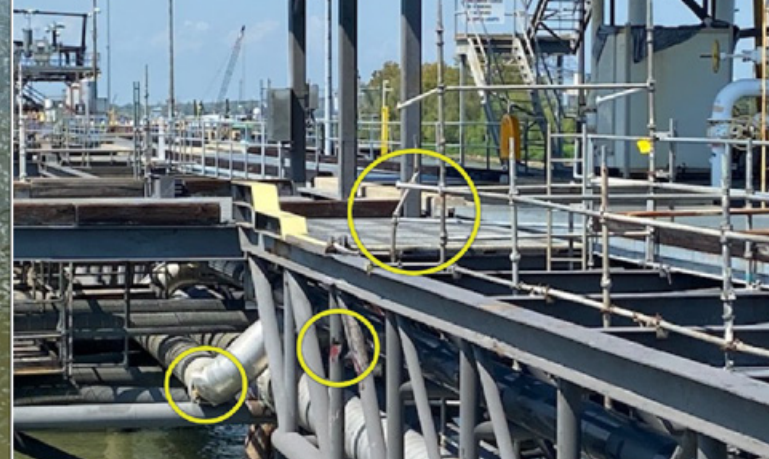
Damage to pier (circled). Left to right: A vertical piling. Insulated pipe, pier support bracing, and railing.
