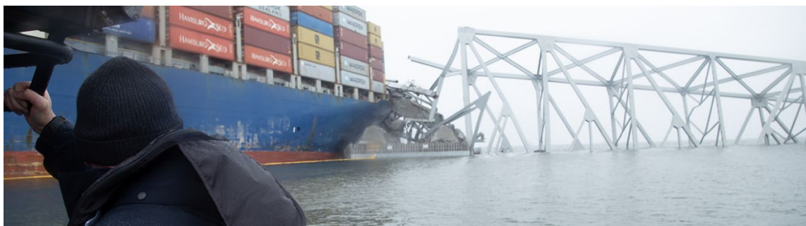
Figure 8. Daniel Walsh, general engineer, studies the starboard side of the containership Dali near its point of impact with the Francis Scott Key Bridge, which resulted in the deaths of six workers who were on the bridge at the time of its collapse.
