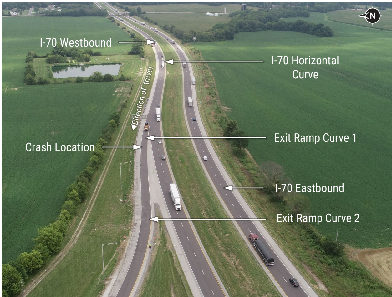
Figure 18. Overhead photo of I-70 and the exit ramp to the Silver Lake Rest Area in the vicinity of the crash. Annotations of the horizontal curves on I-70 and the exit ramp leading up to the crash location are included.
