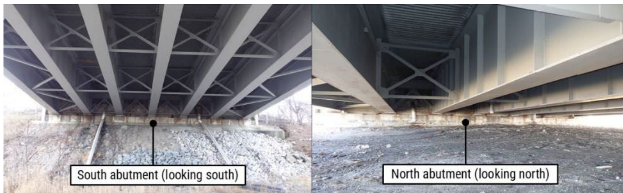
Figure 23. Left to right: South abutment (looking south), and north abutment (looking north). (Background sources: MDTA)
