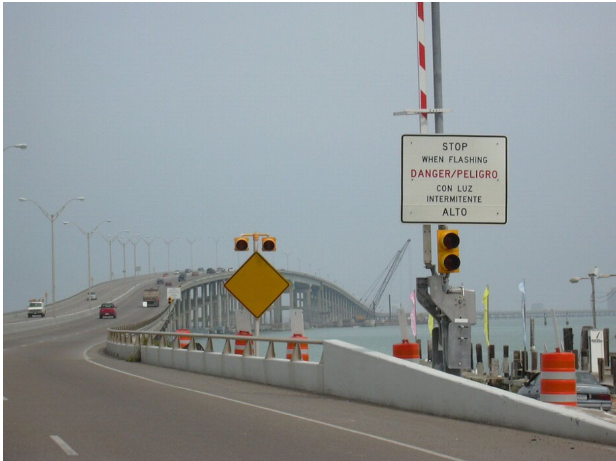
Figure 72. Traffic gates, warning signs, and motorist warning lights installed on the rebuilt Queen Isabella Causeway bridge. (Source: Texas DOT)
