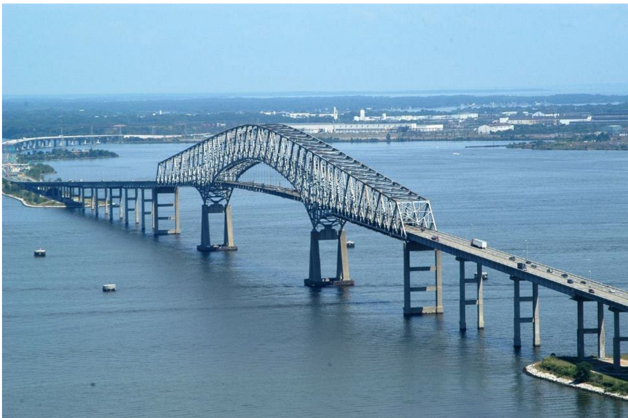
Figure 2. The Francis Scott Key Bridge in 2004. (Source: MDTA)
