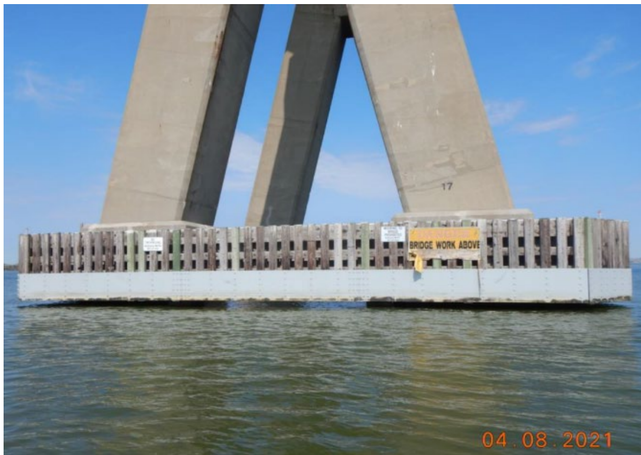
Figure 31. Pier 17, looking north, showing the fender system. (Source: MDTA)
