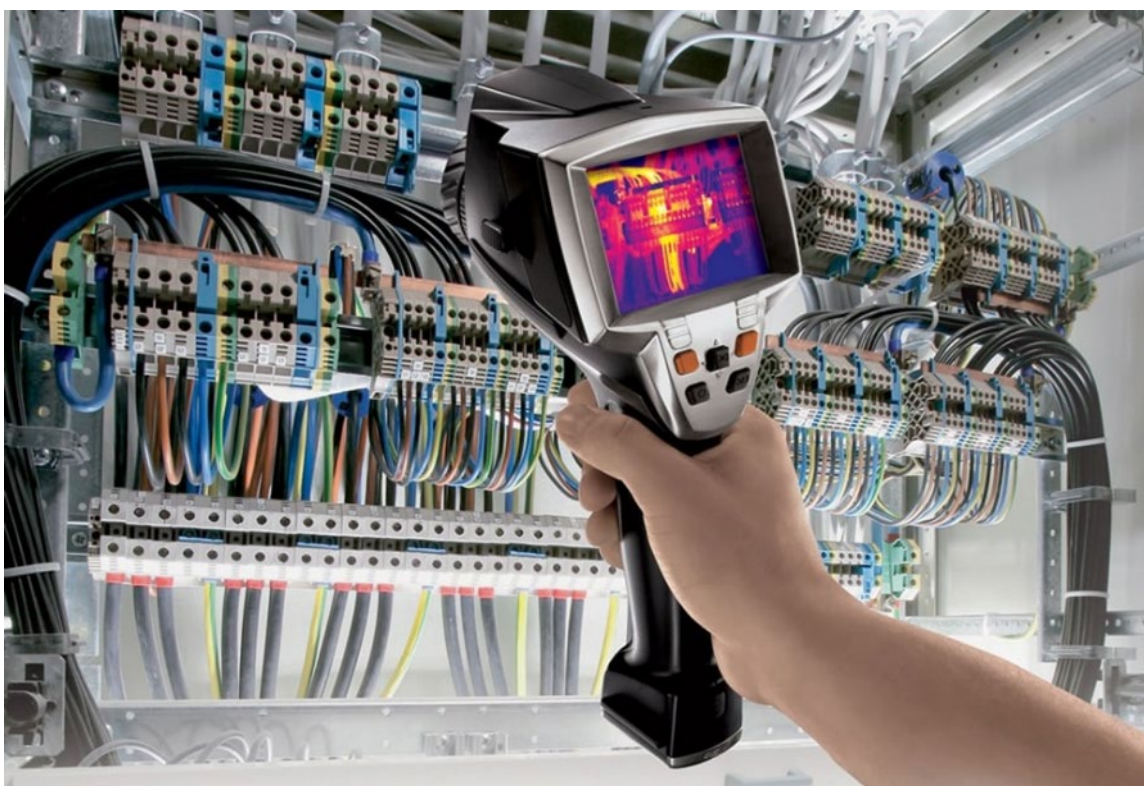
Figure 66. Exemplar infrared thermal imaging camera being used on control circuitry. The lighter colors indicate warmer temperatures. (Source: ThermoElite Inc.)
