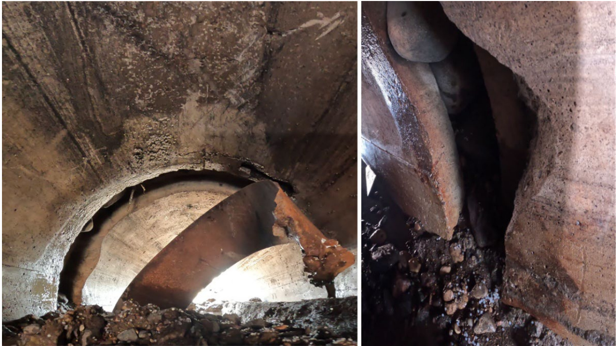
Figure 26. Interior of west culvert looking north ( left ) and west ( right ). (Source: CPKC.)
