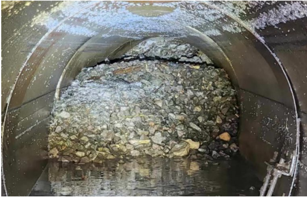
Figure 23. East culvert upon examination and before cleanout.
