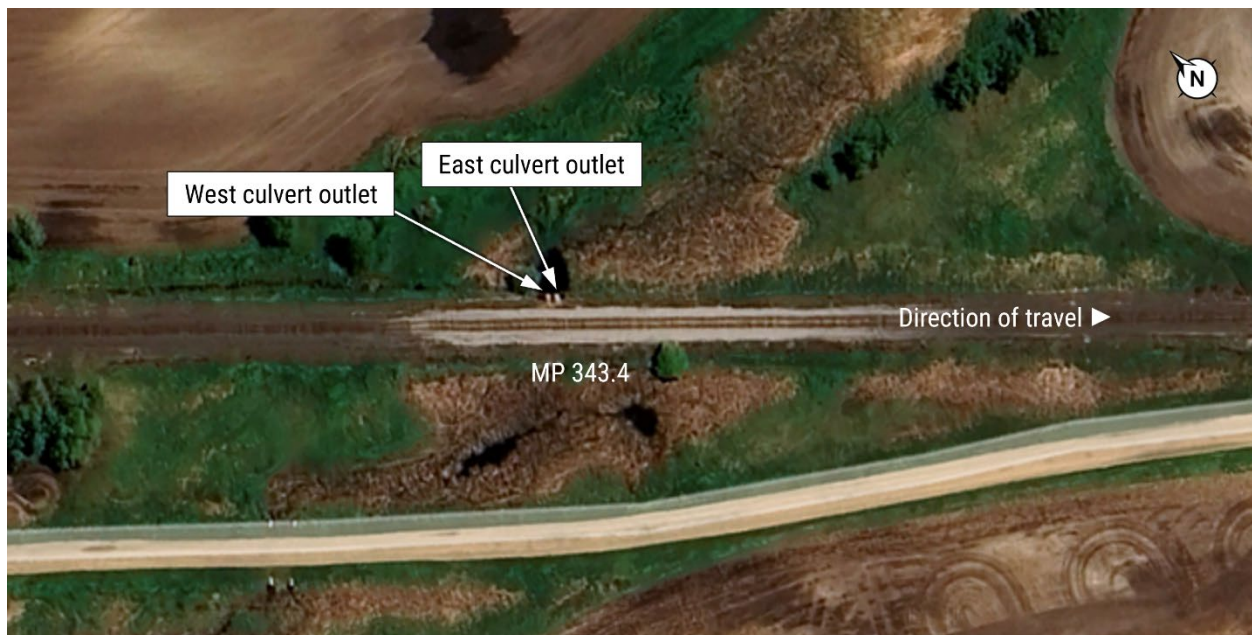
Figure 6. Aerial image of derailment location. (Source: Google Earth).
