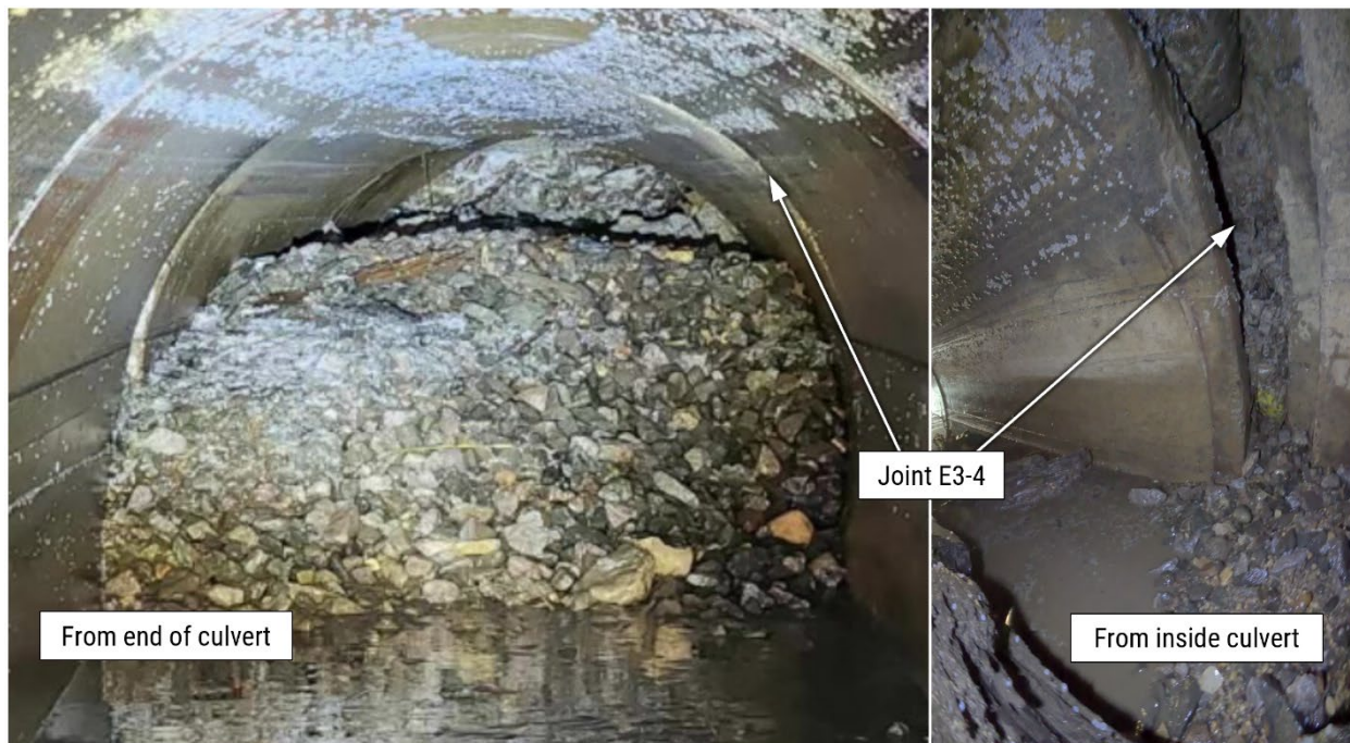
Figure 29. Joint E3-4 viewed from the end ( left ) and inside ( right ) the east culvert.
