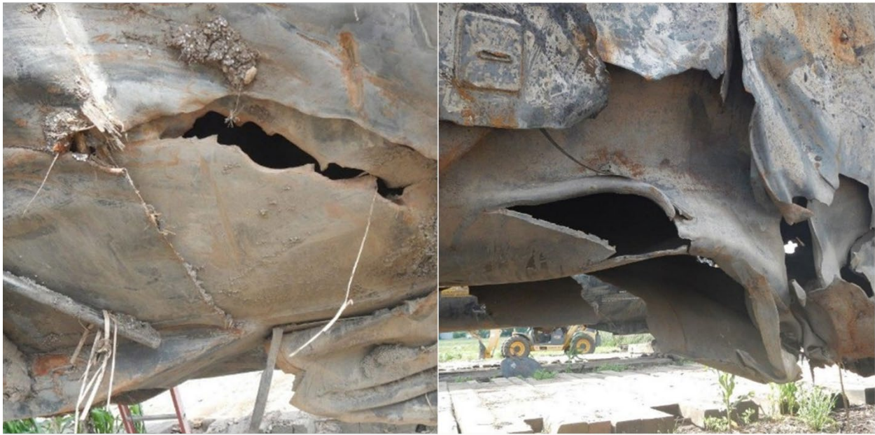
Figure 20. Tank car (63) CTCX300358 shell tears.
