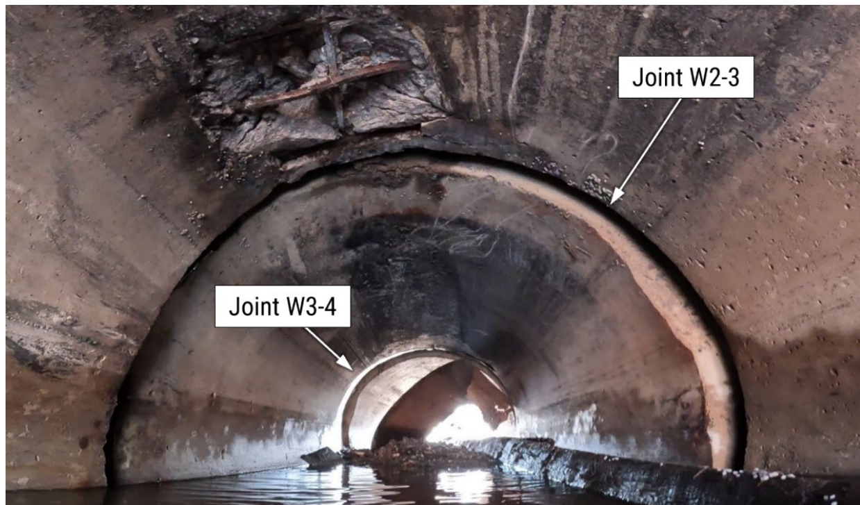
Figure 25. Interior of west culvert looking north. (Source: CPKC.)
